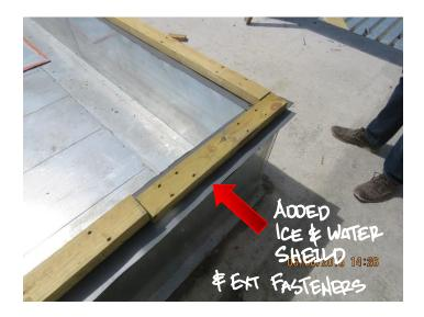
Treated wood blocking requires an ice and water shield separation between the wood and the frame and the use of exterior coated or stainless steel fasteners.
